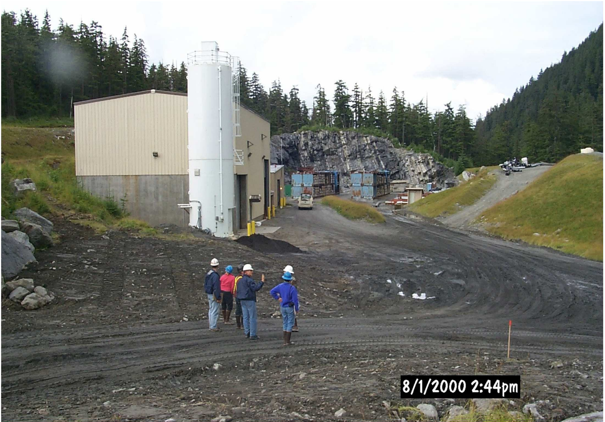
Greens Creek Mine – Upper Water Treatment Building
