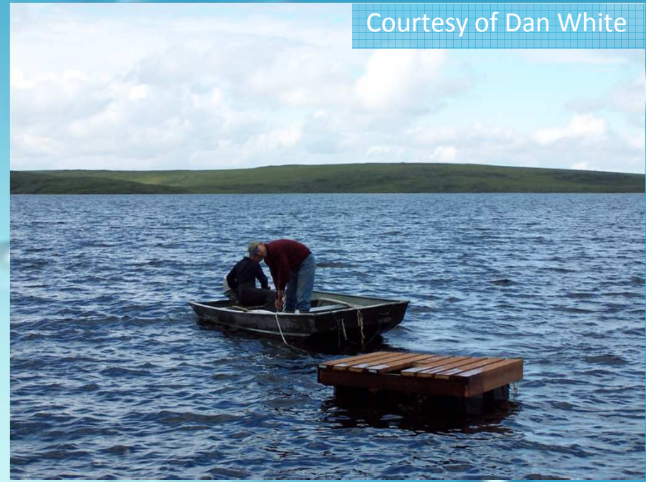
Submersible pump below floating deck
